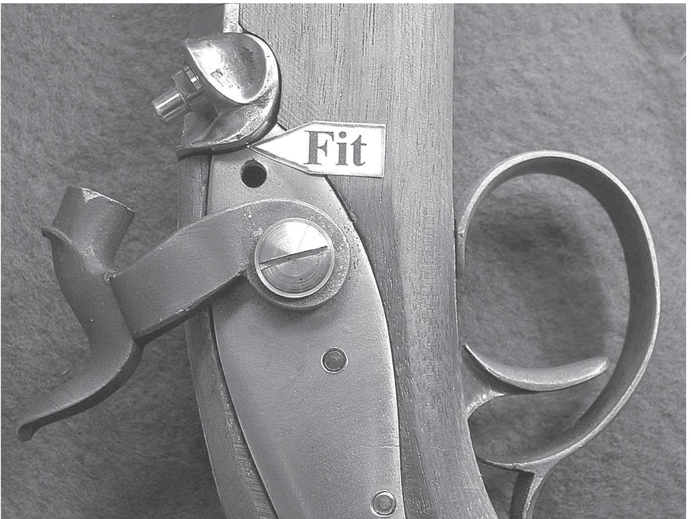
*Figure 6 – Lock needs to be “fit” to snail of breech for proper hammer throw.*
